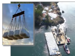
Burrows Island – Barge Removal of "Super Sack" Contaminated Soil
